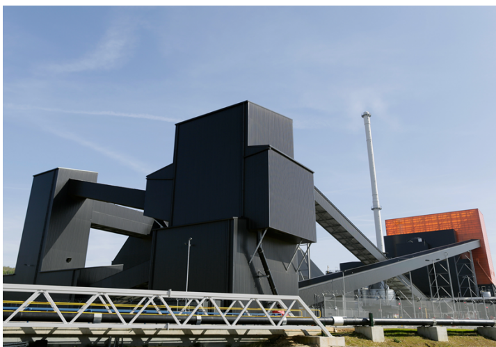
EON, Blackburn Meadows biomass CHP
